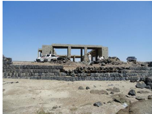
Damaged wave protecting wall
