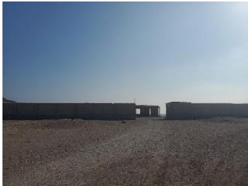
The landing site wall
