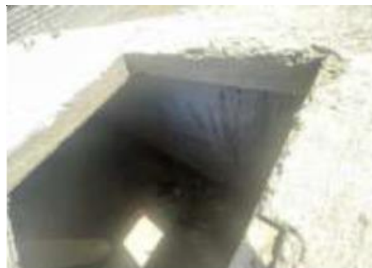
Incomplete underground water tank
