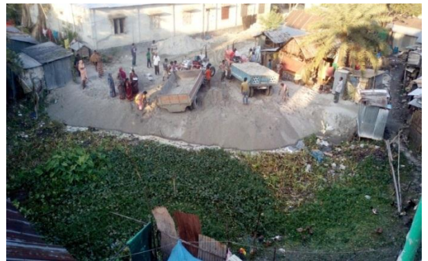
Figure 4.29: Land filling and construction of footpath.
