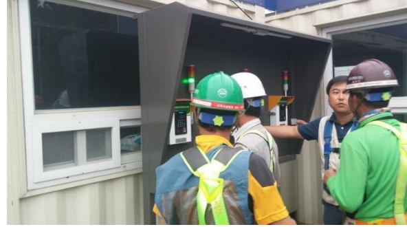
Construction Workers Swiping their RFID Cards
